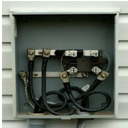
Step 2a Hi-Lug Ground Installation
